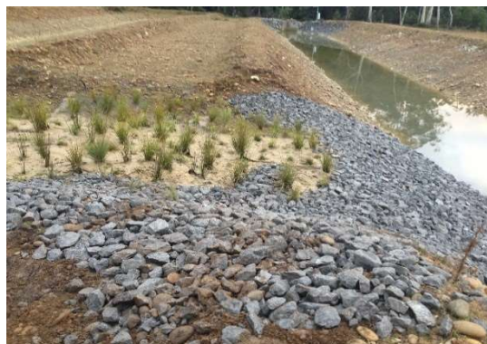
Photo 2: Eastern Settling Pond
