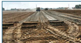
from this reaction further dries wet soils. The reaction with water occurs even if the soils do not contain significant clay fractions. When clays are present, lime's chemical reactions with clays increase the moisture-holding capacity of the soil, which reduces free liquids and causes further drying.
