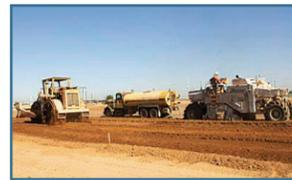
After initial mixing, the calcium ions (Ca++) from the lime migrate to the surface of the clay particles and displace water and other ions. The soil becomes friable and granular, making it easier to work and
