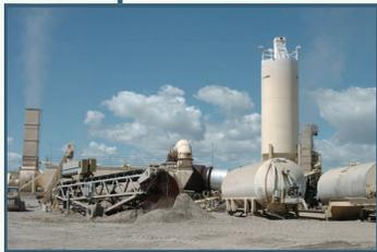
Asphalt plant utilizing dry method of application. Storage containers onsite hold the hydrate, asphalt and burner fuel.
