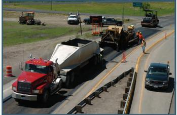
The paver spreads the asphalt, a series of compacting rollers follows.
